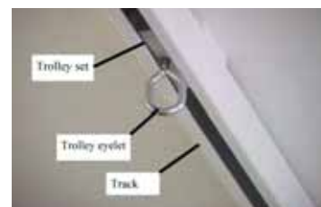
Figure 7A - Photo showing the lift trolley that is installed along the inside of the track. The eyelet of the trolley connects to the hook of the lift in one of several ways.
